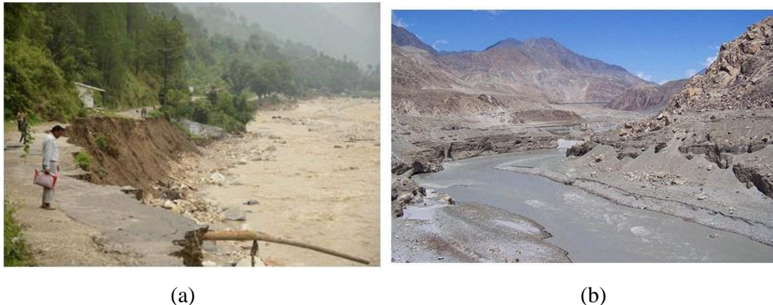
Fig. 2.8 Stream Bank Erosion
